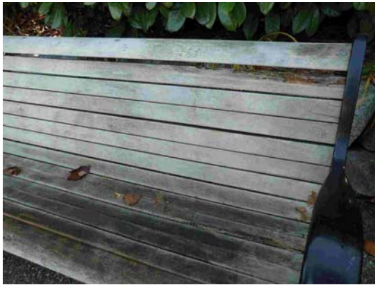
Rotting bench planks need replacement.
