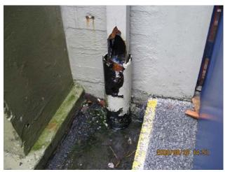
8/28 (VD): Overflowing broken downpipe at the Forum.
